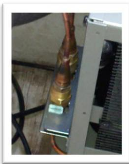
Next step was to carefully engage the two quick connect fittings on the tubing from the evaporator to the condenser. Just make sure they are not cross-threaded and quickly tighten them. A small hiss can be heard. The unit is now ready for the electrical.
