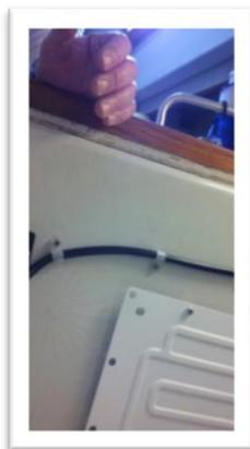
The 16" x 8" x 10" evaporator plate only has a few placement options. I chose to keep the large part of the plate near the galley and away from the hull side which is the warmest part of the box. The plate easily screws into the box with stand-off pegs. A thermostat switch is also installed very close to the front of the box with wires being attached neatly with clips. The thermostat is cleverly rounded to fit in the curved corner of the ice box.
